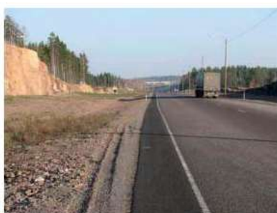
Figure 4.21. Recoverable ditch shapes: 1:4 fore slope, rounded bottom and 1:2 back slope. (Photo, HUT)
