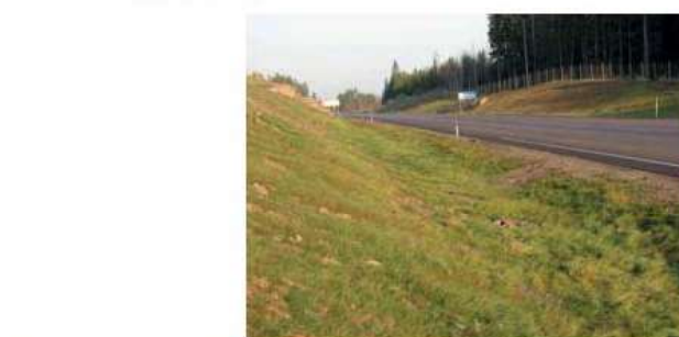
Figure 4.22. Recoverable fill slope; bottom of the ditch is rounded, no hazardous obstacles in fill slope. (Photo, HUT)
