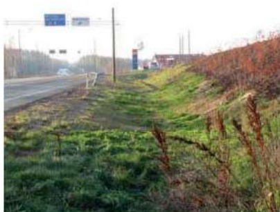
Figure 4.21. Recoverable ditch shapes: 1:4 fore slope, rounded bottom and 1:2 back slope. (Photo, HUT)
