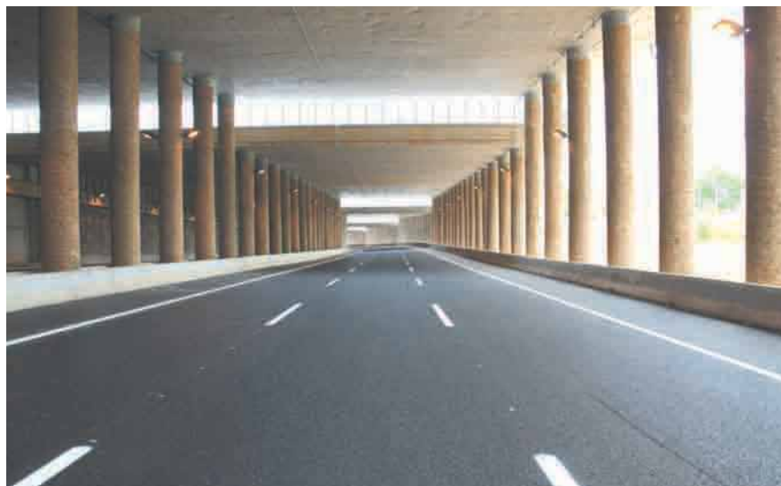
Interior de la cobertura de Can Tries.
