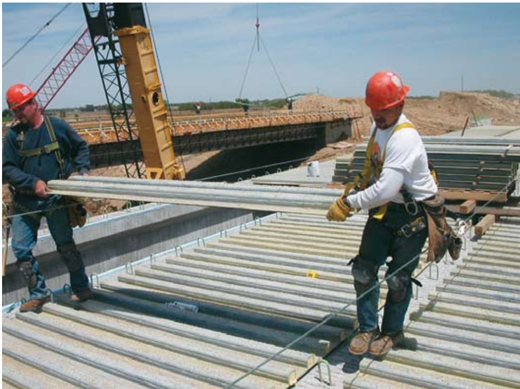
Fig. 21. FRP SIP/reinforcement panel being placed.
