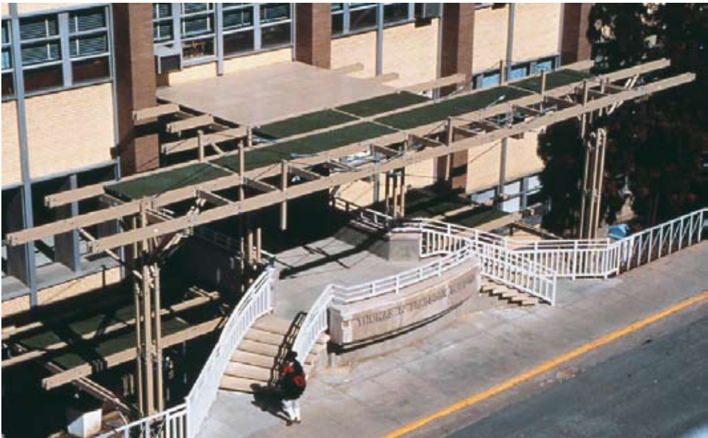
Fig. 4. Cable-supported FRP building system.
