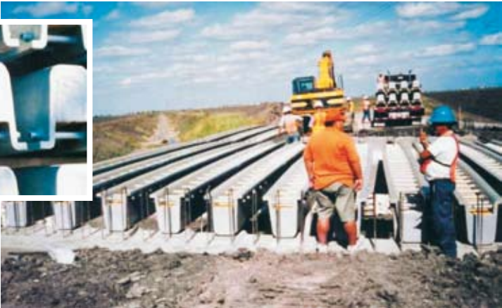
Fig. 12. Molded FRP U-girders installed on abutments (photo: MFG).
