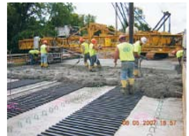
Fig. 23. Pultruded planks as permanent formwork panels.
