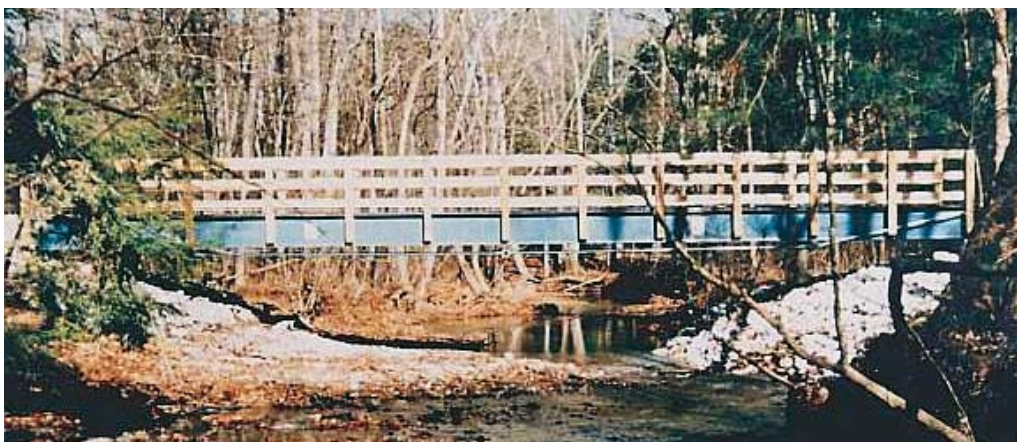
Fig. 6. Hybrid FRP girder bridge with cable (photo: Strongwell).
