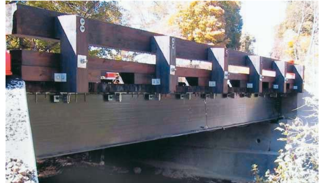
Fig. 9. Installation of FRP Double web pultruded girders on Rt. 601 bridge (photo: Strongwell).
