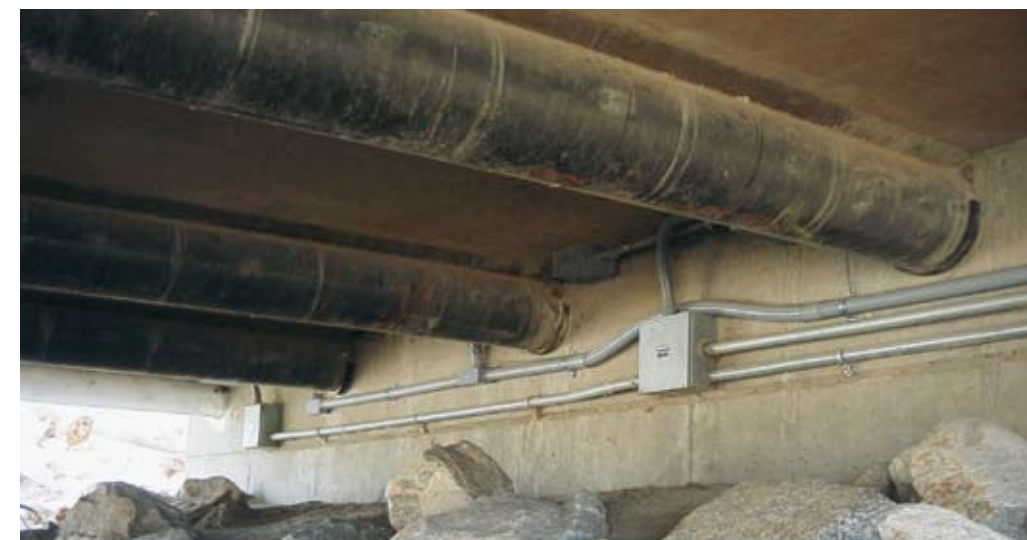
Fig. 20. Hybrid FRP tube/concrete girders in California.
