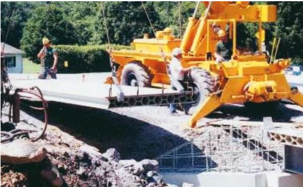
Fig. 17. Installation of Superdeck in 1997 (photo: Creative Pultrusions).
