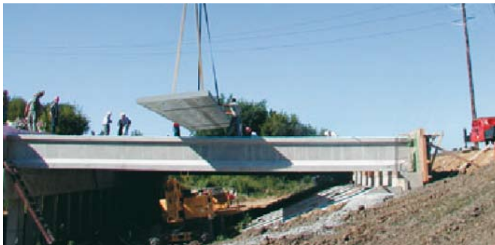
Fig. 19. Installation of FRP deck panels on PC girders (photo: Martin Marietta Composites).
