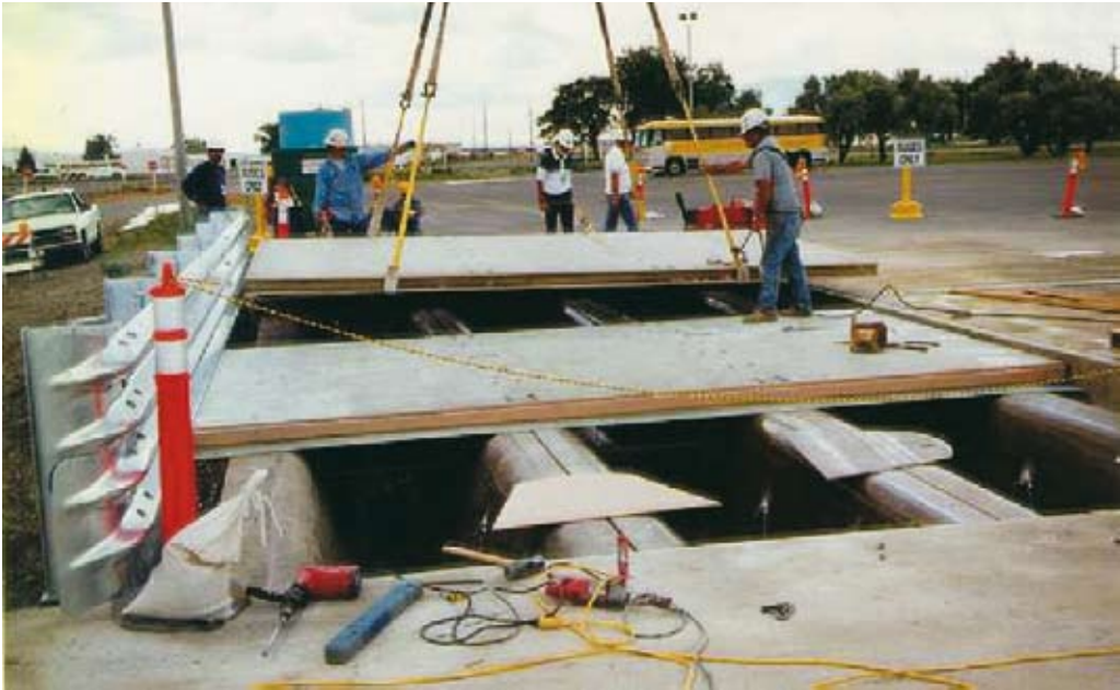
Fig. 14. First FRP deck panel installed in the USA in 1995 (photo: Martin Marietta Composites).
