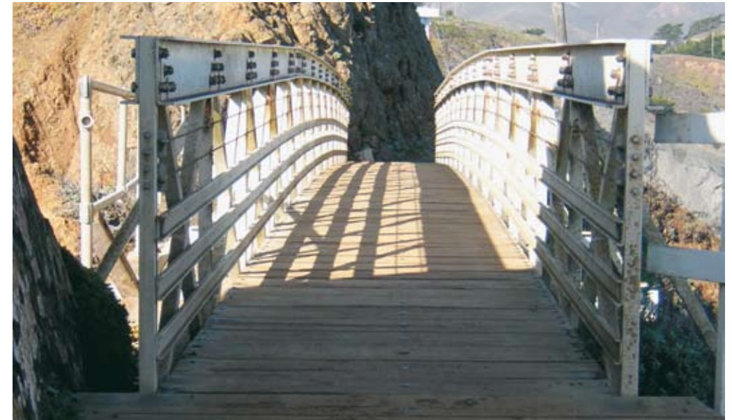
Fig. 2. End view of pultruded truss bridge.
