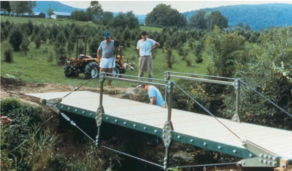
Fig. 3. Prestek® Cable supported FRP pedestrian farm bridge (photo: ETTechnics).
