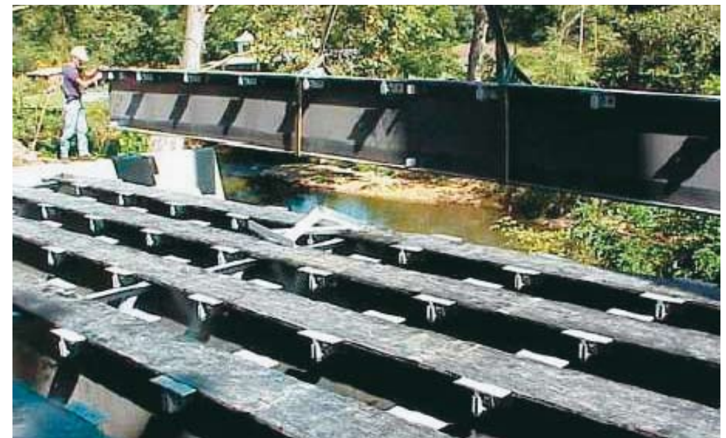
Fig. 10. Timber guardrail and deck on Rt. 601 bridge (photo: Strongwell).
