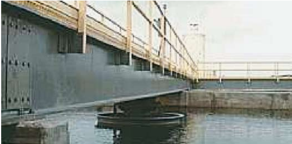
Fig. 5. FRP I-girder bridge (photo: Strongwell).
