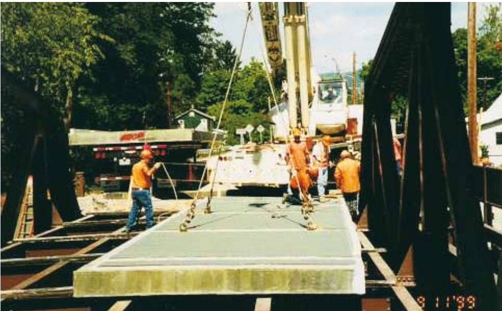
Fig. 15. Installation of molded panels on steel stringer bridge (photo: J. O'Connor).
