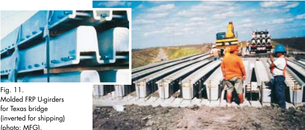
Fig. 12. Molded FRP U-girders installed on abutments (photo: MFG).
