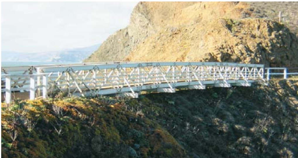
Fig. 1. 24 m long FRP pedestrian truss bridge.
