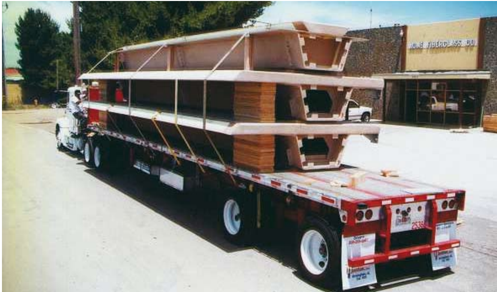
Fig. 8. Molded trapezoidal girders (with FRP deck) for the TECH 21 bridge (photo: Martin Marietta Composites).
